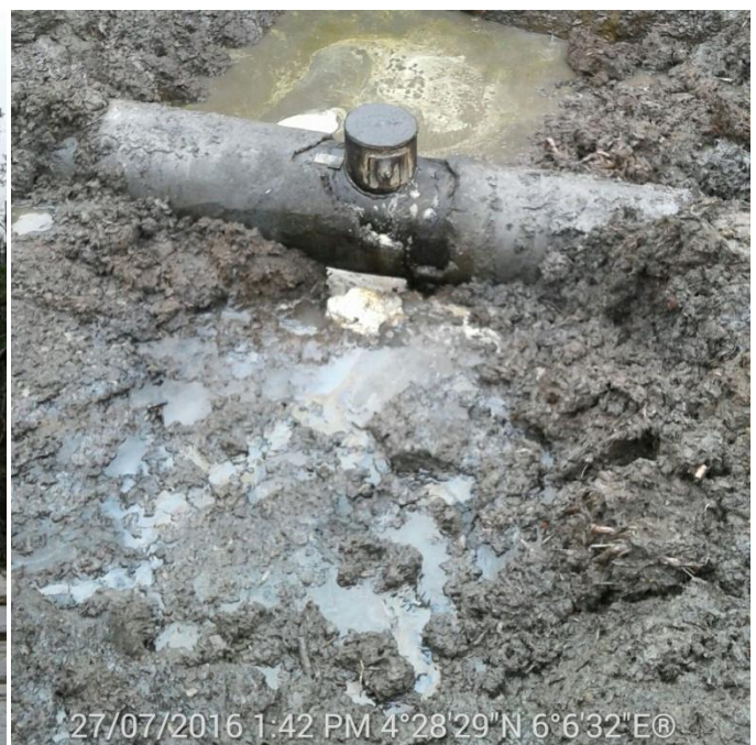
Fig D: Incident Facility during repair.
